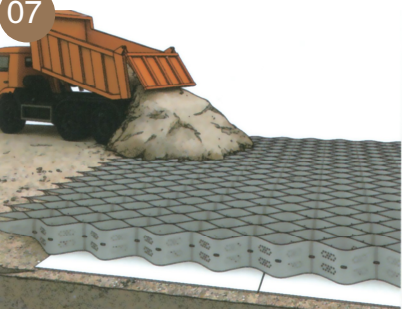
Fill GEOCELL with the filler.
