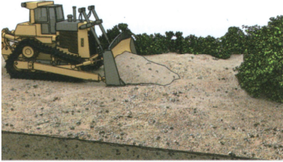
After grading the ground, remove the plant roots and stones.
