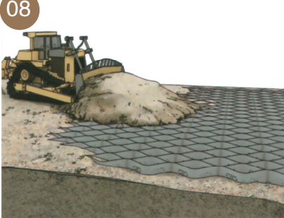
Spread soil and filler evenly using the equipment
